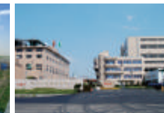
TBR Plant in Xiasha
