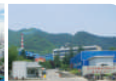
Bias Tyre Plant in Xinanjiang
